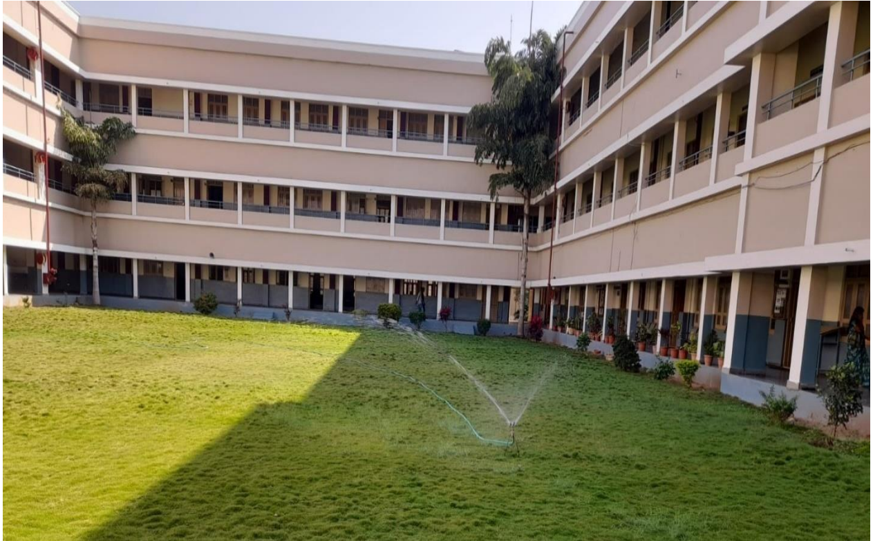
Fig7: Sprinkle Water system at lawns in the campus
